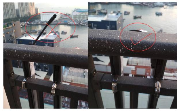
3 Each light should use exc's exclusive end cap, The end cap should be fixed on the end port of light fixture. Or use structural glue/silica to cover the female hole. Remember wrap insulating tape (in case structural glue flows out before solidification).
