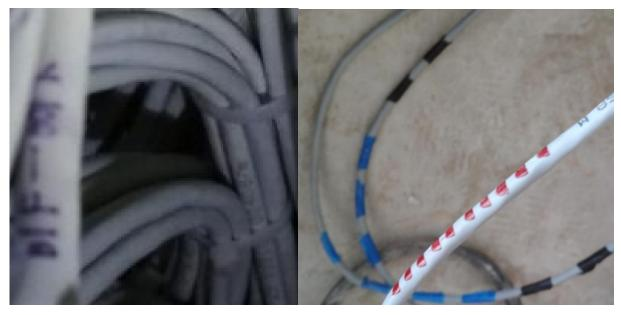
5 It is forbidden that strong and weak electricity go through the same line slot or use one wire tube. The bridge frame of strong electricity and weak electricity must be more than 35 cm apart. The signal line and AC power line must be placed separately and strictly prohibited in parallel. Also not bound together. if must need in parallel method, Please use metal casing , casing spacing greater than 10 cm.
